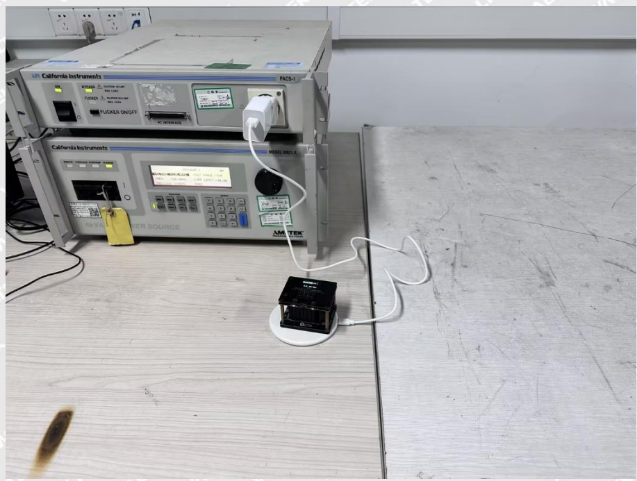
Harmonic/Flicker Test View
